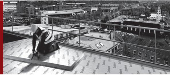
Xtratherm FR/TP Thermal Ply is a composite insulated panel of Xtratherm Polyisocyanurate core with a composite foil face, bonded to 6mm WBP grade plywood. FR/TP is designed to provide high levels of thermal insulation and decking in one operation for new and refurbishment flat roof applications.
