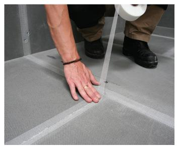
A gap of about 4mm should be left between the edge of the boards and the wall. Next, fill the gap with a visco-elastic adhesive such as Multibond to eliminate the possibility of flanking sound happening there.
